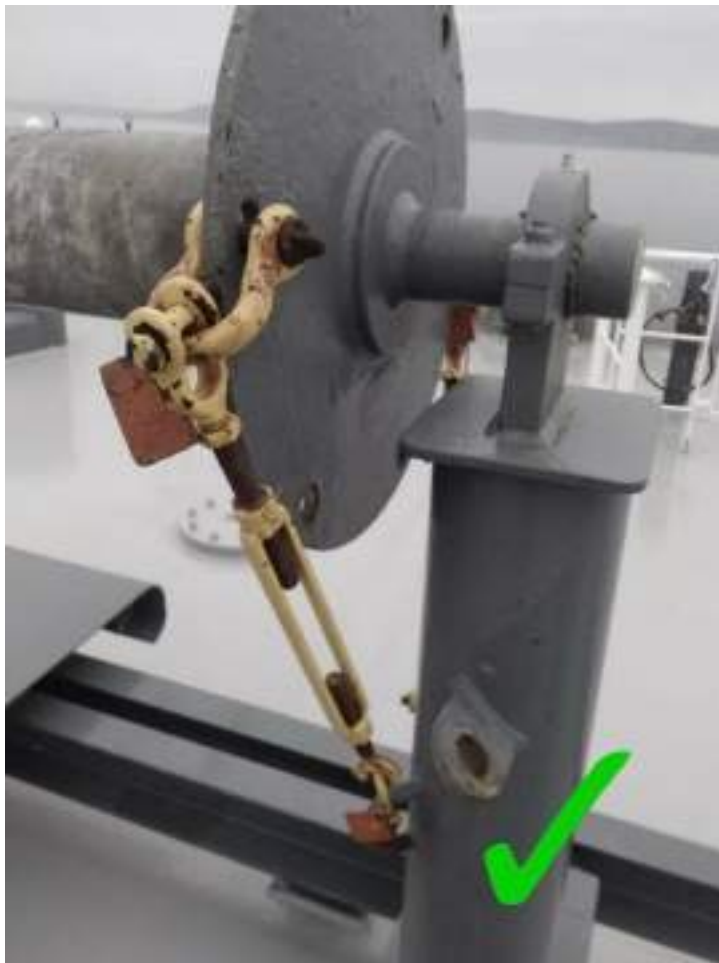
Showing mechanically secured winch reel.
