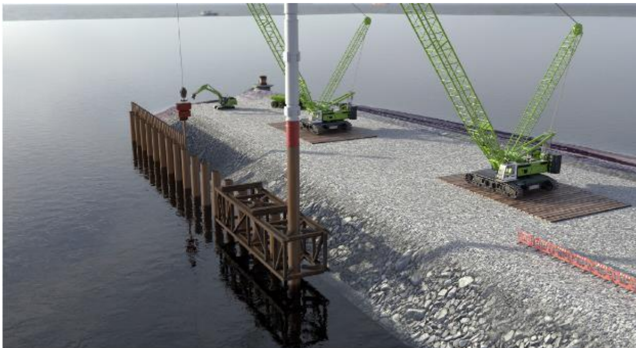
Figure 2-4 Installation of the piles
