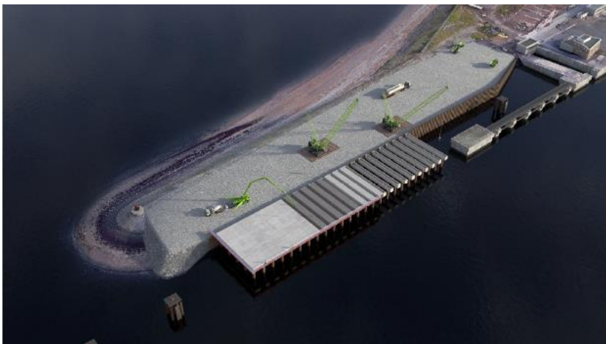
Figure 2-5 Placement of the precast beams, omni planks and pouring of the concrete deck
