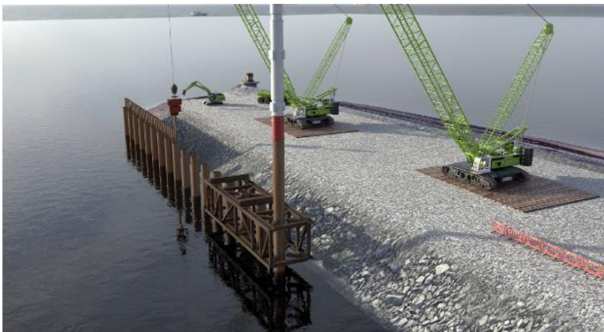
Figure 3-4 Installation of the piles
