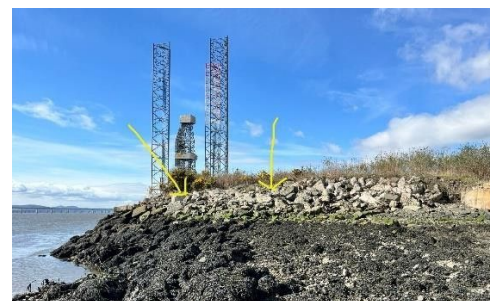
View of rubble pile / rock armour where RS2 (left arrow) and RS3 (right arrow) are located. Also shows the high tide line below
